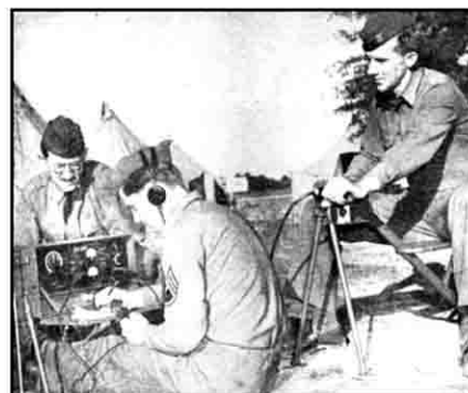
A 1942 US Army photo showing the proper use of the BC-474. Note the soldier on the right turning the generator crank, while the operator receives a message. The soldier behind the radio, an officer, is waiting for the message.
