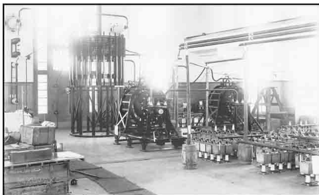
Figure 13—Antenna Coils and Loading Capacitors. (Photo 1929)
