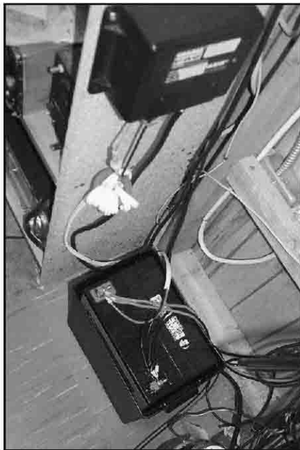
Figure 4—The battery and charger. Note the ferrite choke on the charger leads. The battery is normally covered to enclose its terminals.
